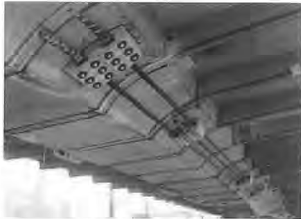
An example of post-tensioning.
